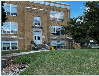
Walnut Street Entrance (Grades 7 & 8)
