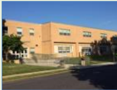
B-Building (Edgewood Avenue)
